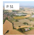
P. 51 Surplus heat integrated into district heating
